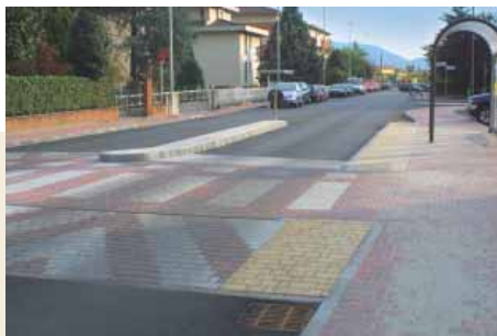
Pedestrian right of way through raised crossing
